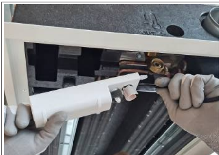
Fig. 26: Dismantling the condensate pump
