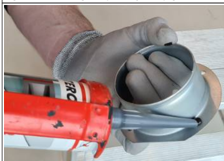
Fig. 21: Sealing the primary air connection spigot
