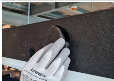
Fig. 20: Removing the primary air spigot
