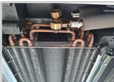
Fig. 16: Insulation as far as the thread
