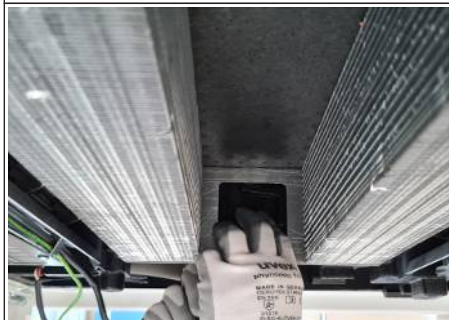
Fig. 22: Removing the primary air cover
