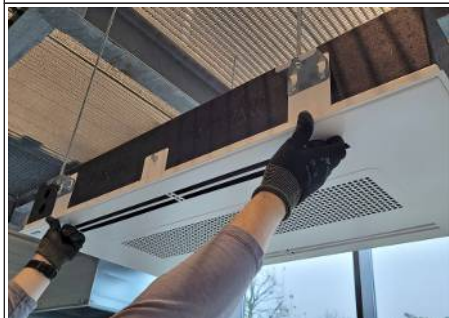
Fig. 7: Opening the design panel
