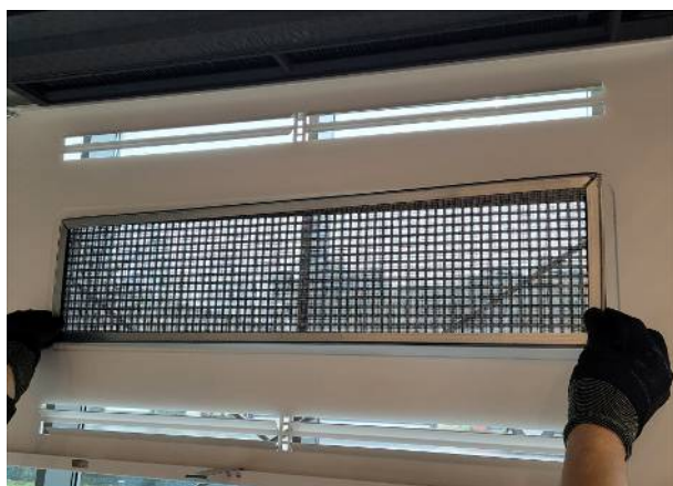
Fig. 24: Remove the filter.
