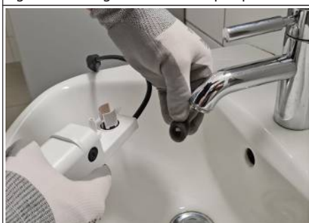
Fig. 28: Cleaning the dirt filter
