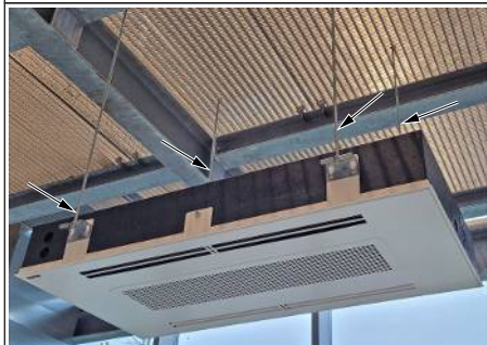
Fig. 6: Unit suspended
