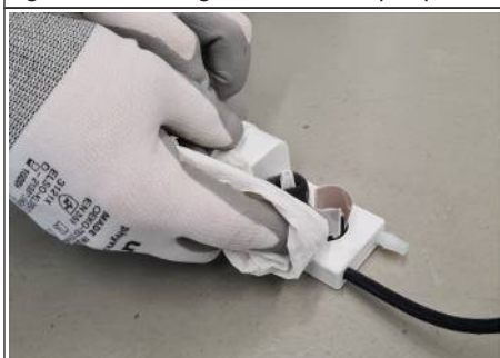
Fig. 27: Cleaning the condensate pump
