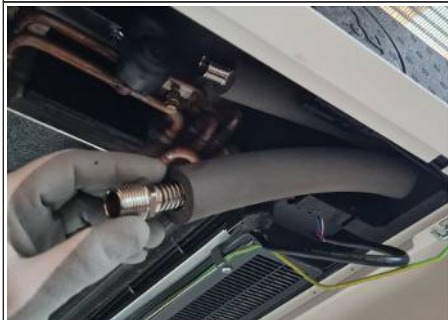
Fig. 15: Flexible corrugated pipes
