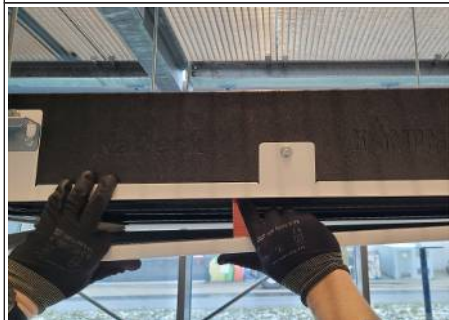
Fig. 8: Pressing in the retaining plate
