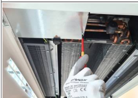
Fig. 17: Opening the electrical connection box
